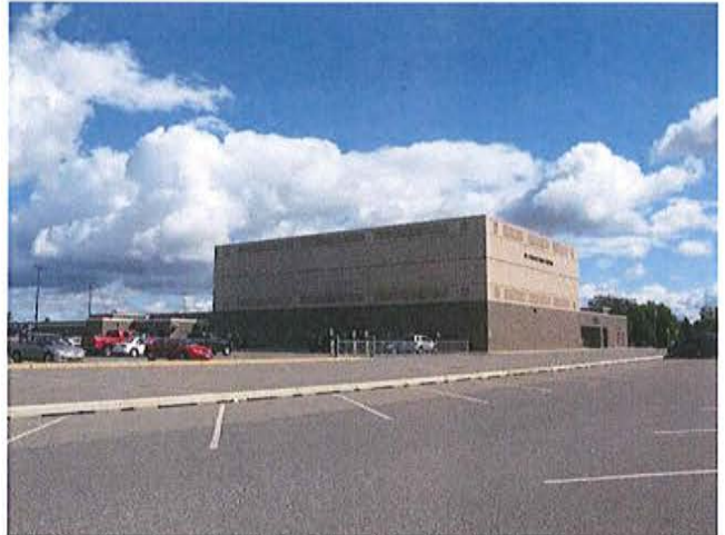
View of St. Francis High School located east of subject Site.
