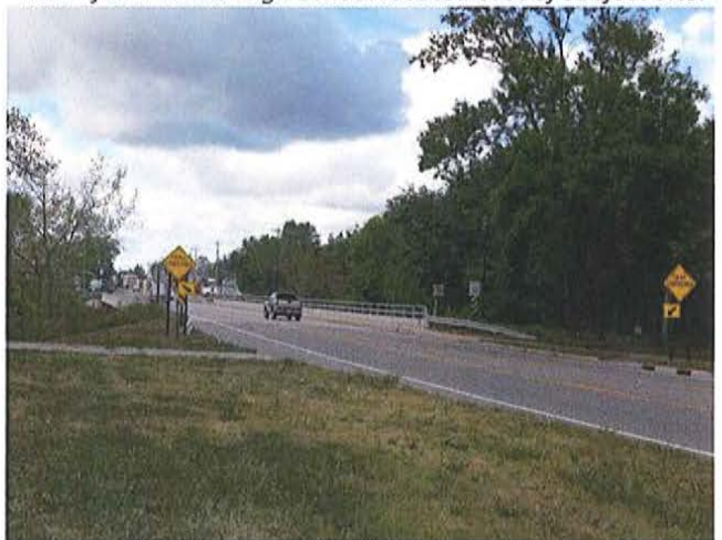
View of Bridge Street looking West of subject Site.
