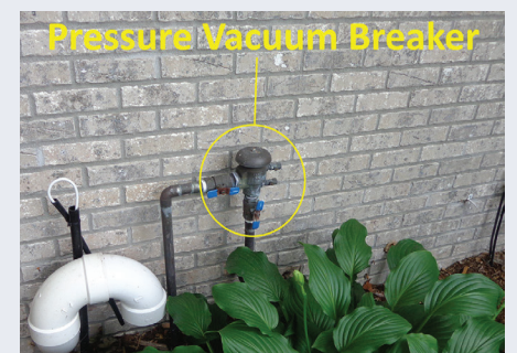
This is not an approved backflow prevention device.
